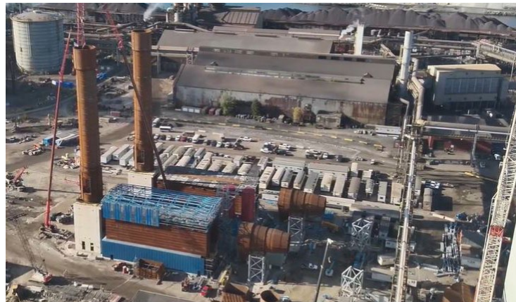
Stacks on Fume Treatment Plants installation
