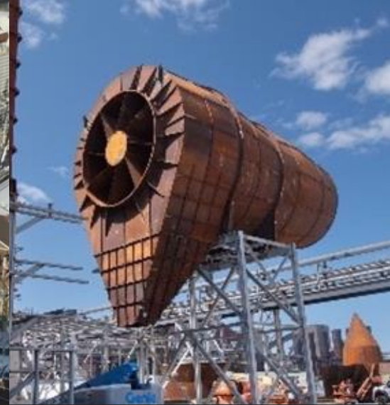
Axial Cyclone installation on Baghouse
