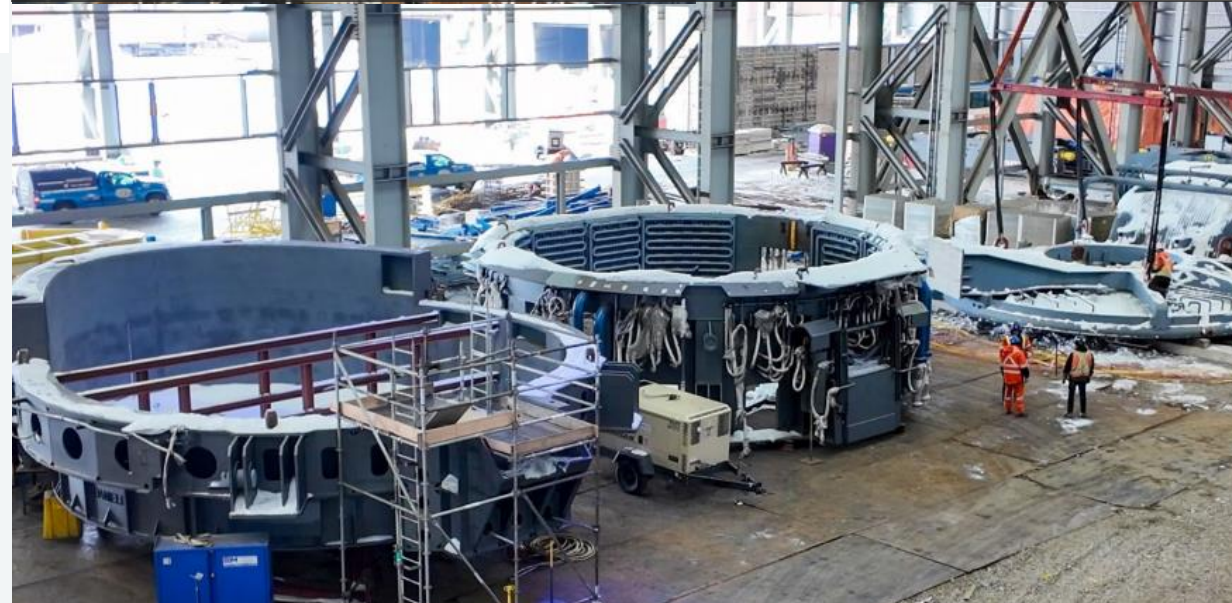
EAF #2 ready for assembly and installation.
