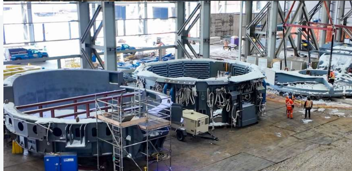
EAF #2 ready for assembly and installation.
